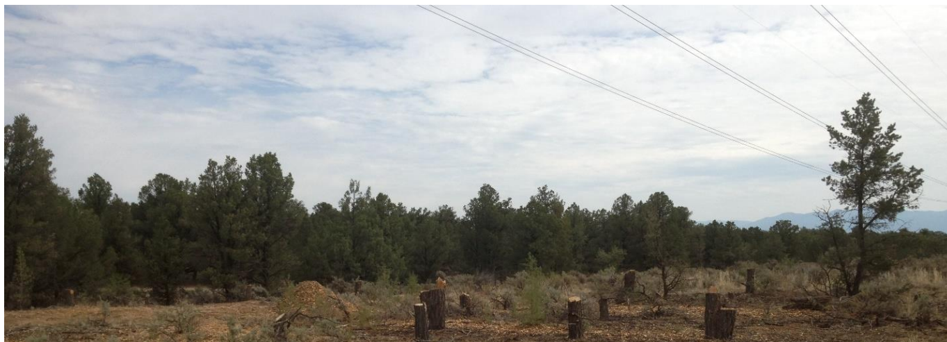
Tri-State Transmission line near Carson © Mary Stuever/NMFD
